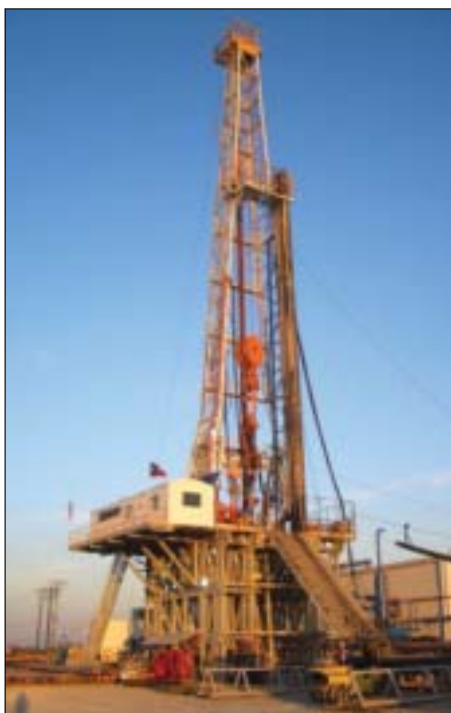
^ Cameron Texas Facility. This facility is equipped with a drilling rig for performing drilling, borehole-measurement and system integration tests. The rig is capable of handling three-joint stands of drillpipe and is equipped with high-volume mud pumps. The rig is mounted on rails for convenient access to different well slots with a wide variety of directional wells that can be used for both openhole and cased-hole tests.
